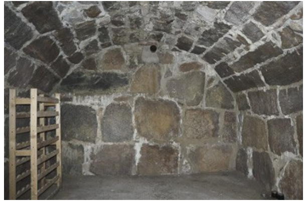
Blick in den Erdkeller
